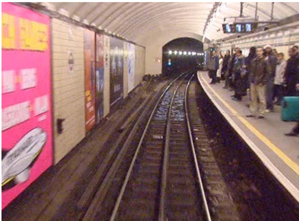
Photograph showing curved platform at Kings Cross 4
