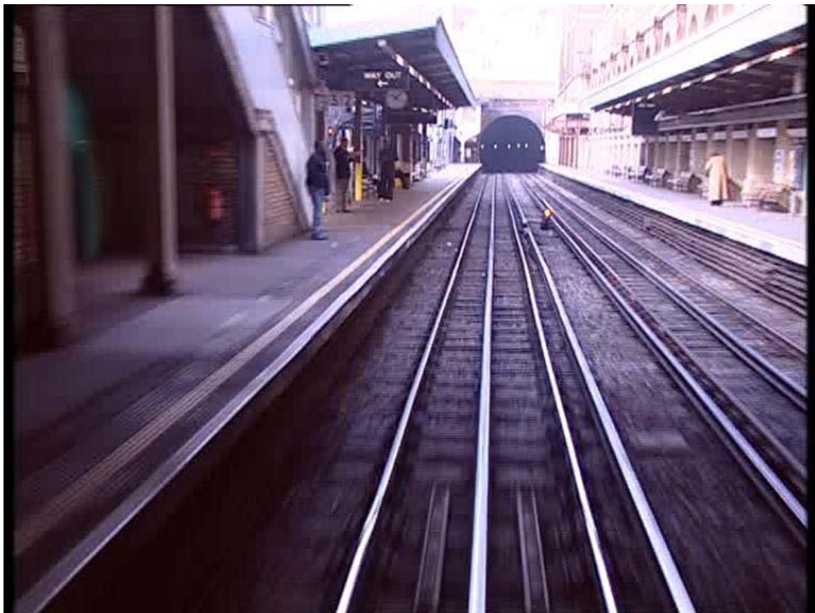
Photograph showing straight platform at Barbican 2
