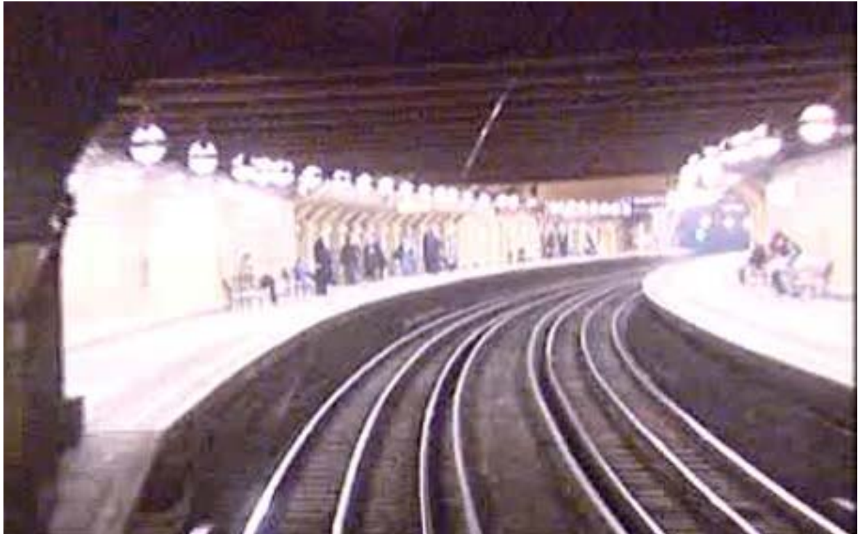
Photograph showing severely curved platform at Great Portland St 5
