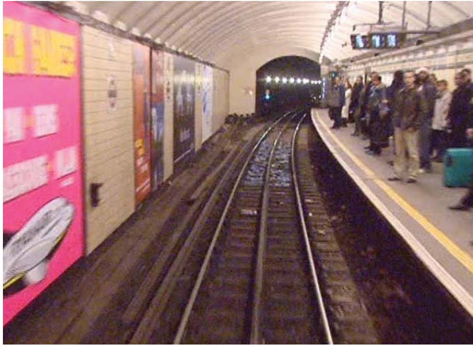
Photograph showing curved platform at Kings Cross 15
