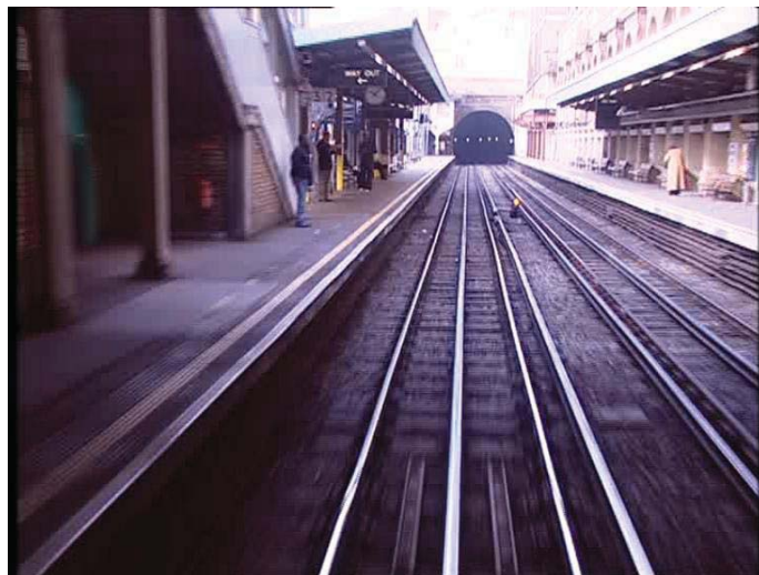
Photograph showing straight platform at Barbican 13
