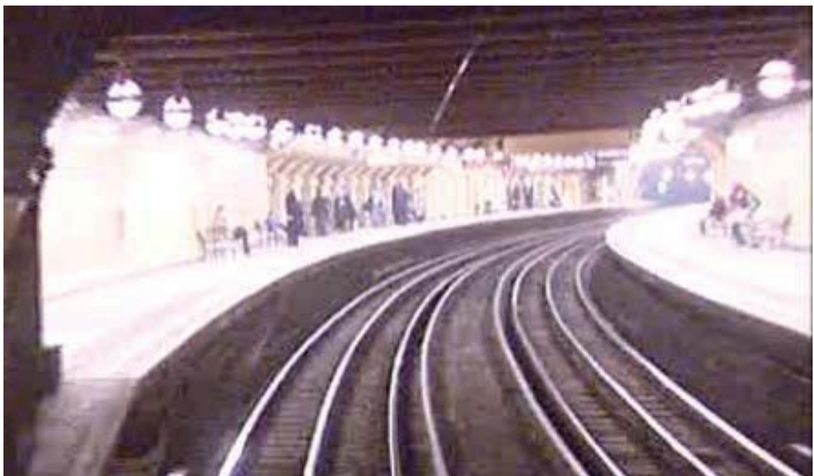
Photograph showing severely curved platform at Great Portland St 16
